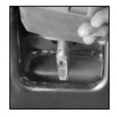
If you look under the receiver you will see the locking portion (clip) of the pin coming through the bottom hole in the receiver.
